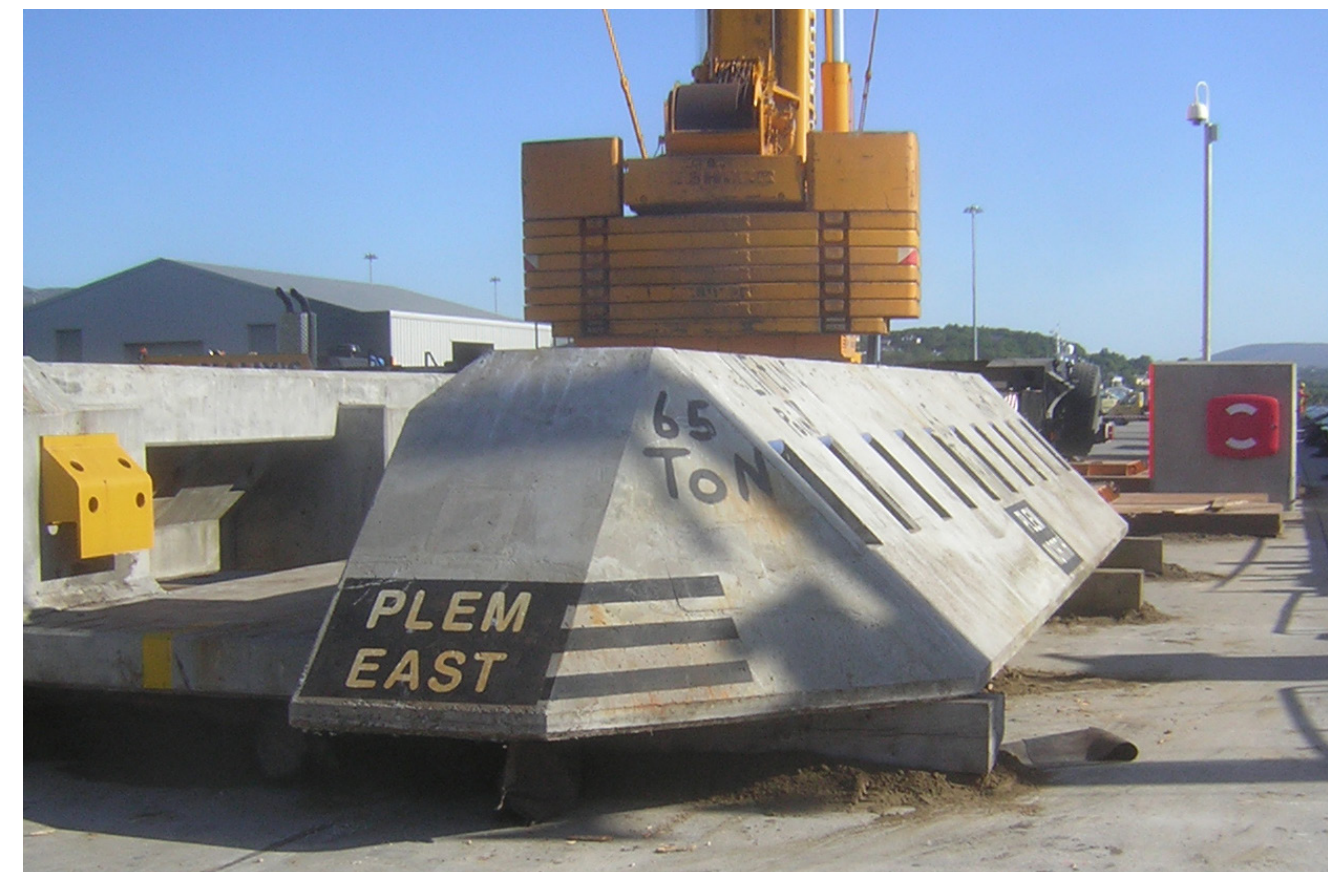
fig. 06/ sand used to level the ground due to presence of drainage channel
