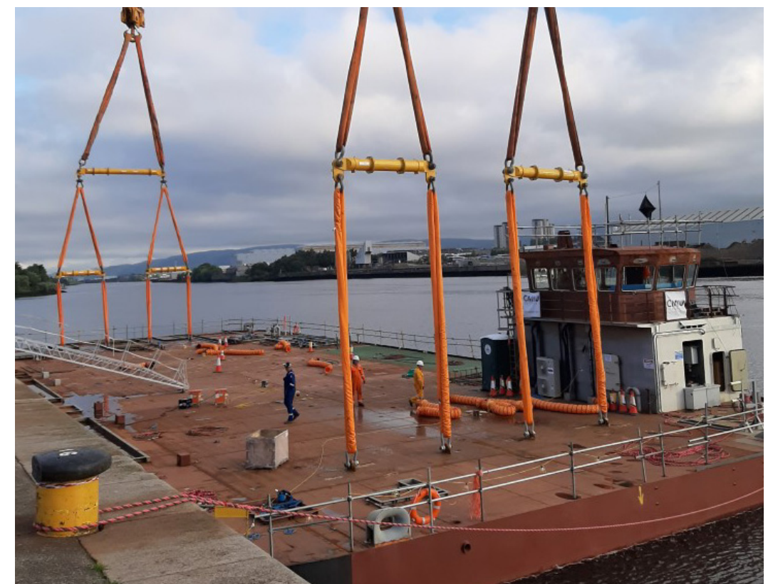
fig. 17/ spreader beams as used in a complex rigging arrangement
