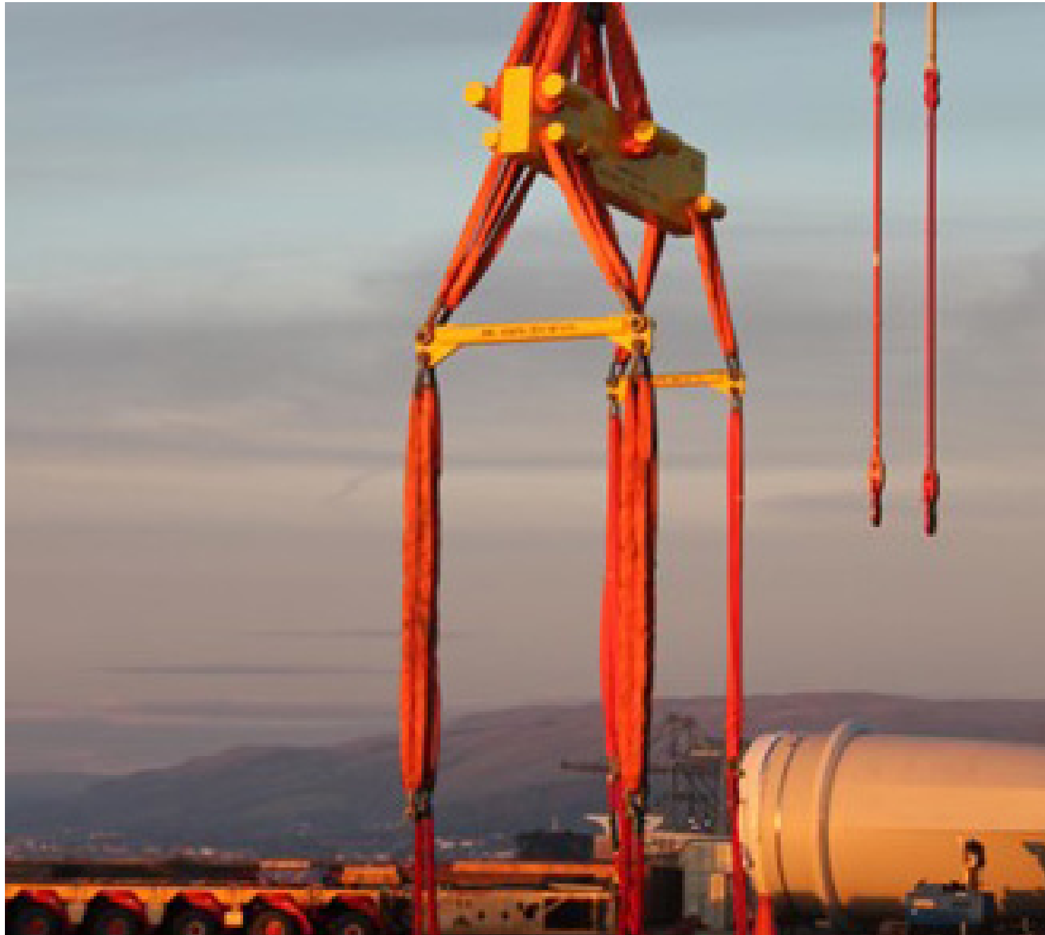
fig. 21/ lift beam and spread beams in use
