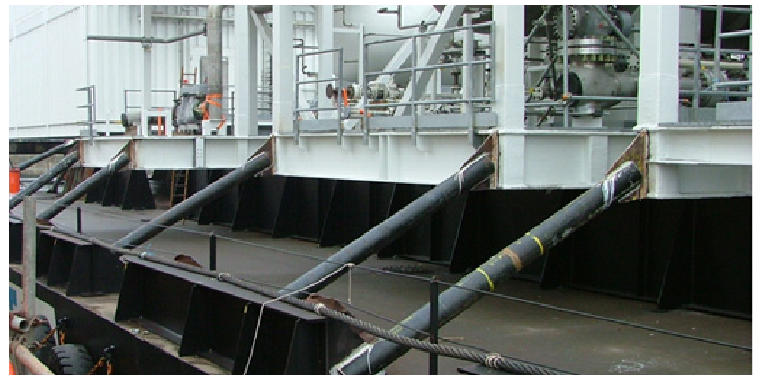
fig. 7/ offshore modules with roll bracing aligned with primary structure
